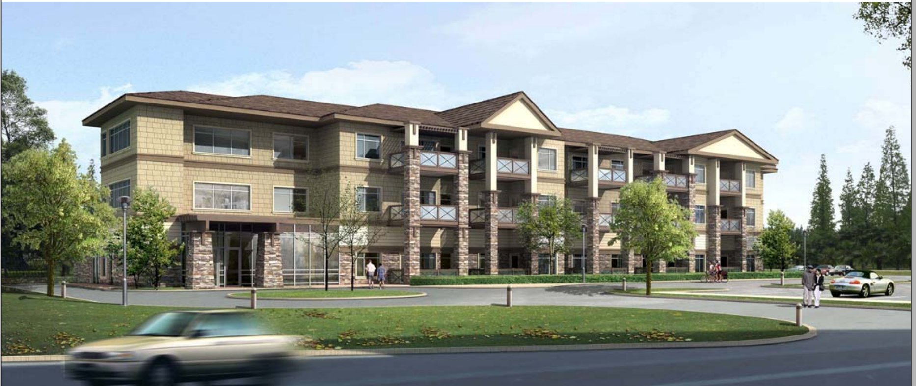
Gimli West Apartments. Affordable not-for-profit rental housing
